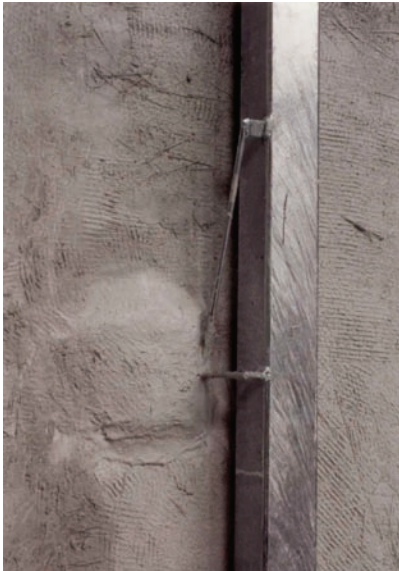
Figure 3: Gravity anchor
